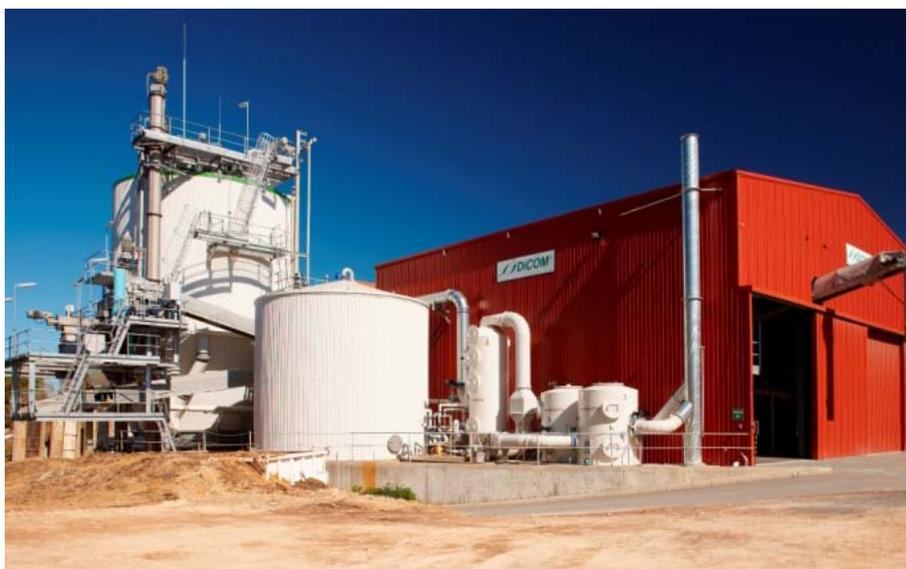
Fig 4 – WMRC Stage 1: bioconversion vessel, water storage tank, odour control system and material recovery facility (MRF) shed. Completed December 2008.
