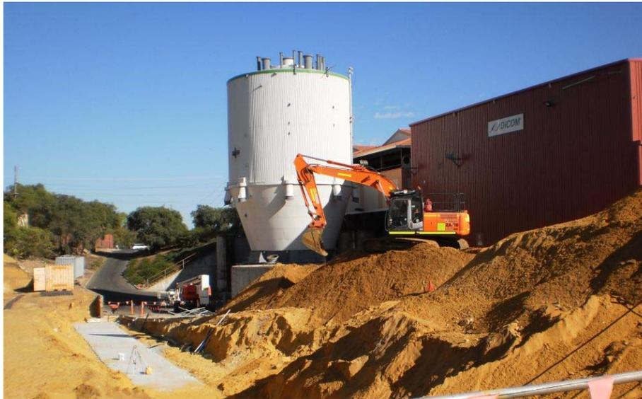
Fig 1 – WMRC Stage 2: bioconversion vessel with all ancillary equipment dismantled. Civil works in progress April 2011
