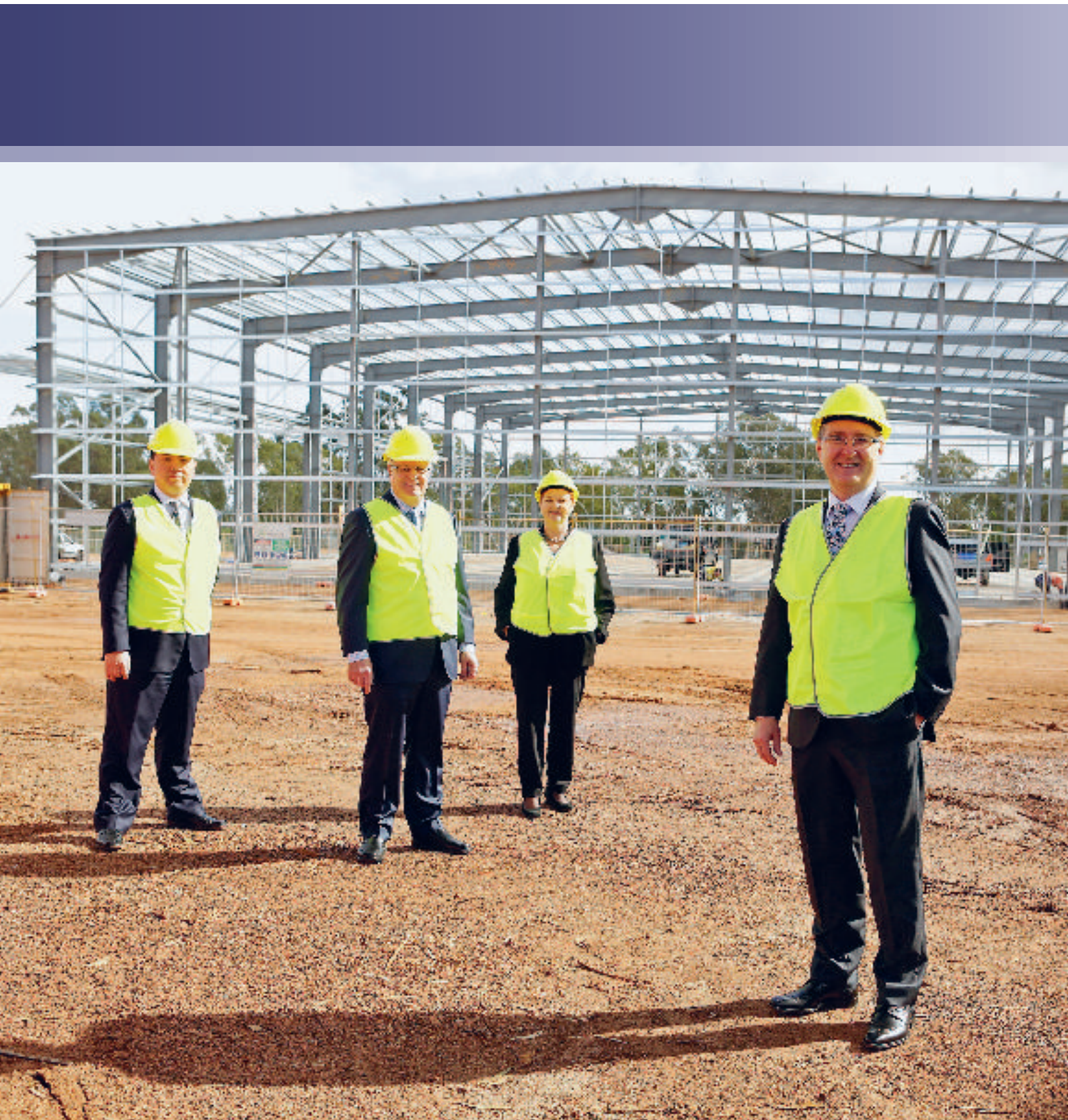
Commercial and Industrial Waste Sorting Facility under construction – June 2016
